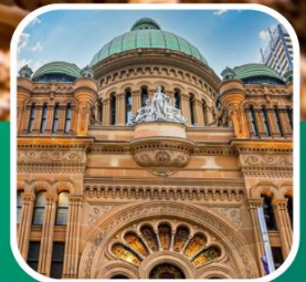
QUEEN VICTORIA BUILDING
