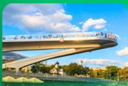
Floating Bridge Moscow
